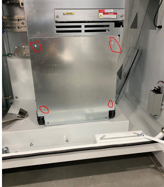
Figure 4-7: Screws at the heatsink fan airway cover.
