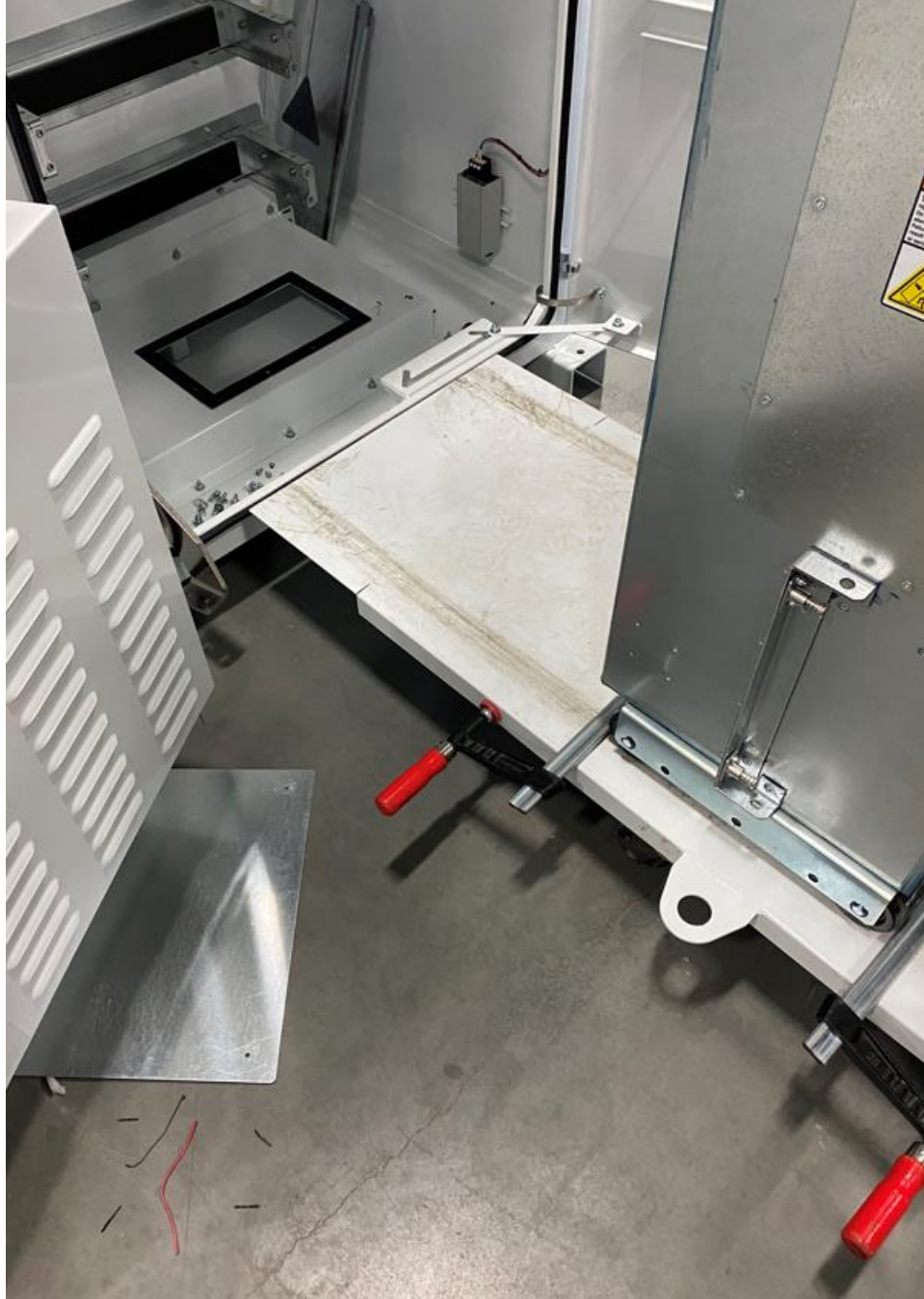
Figure 4-12: Pushing in new module into the enclosure
