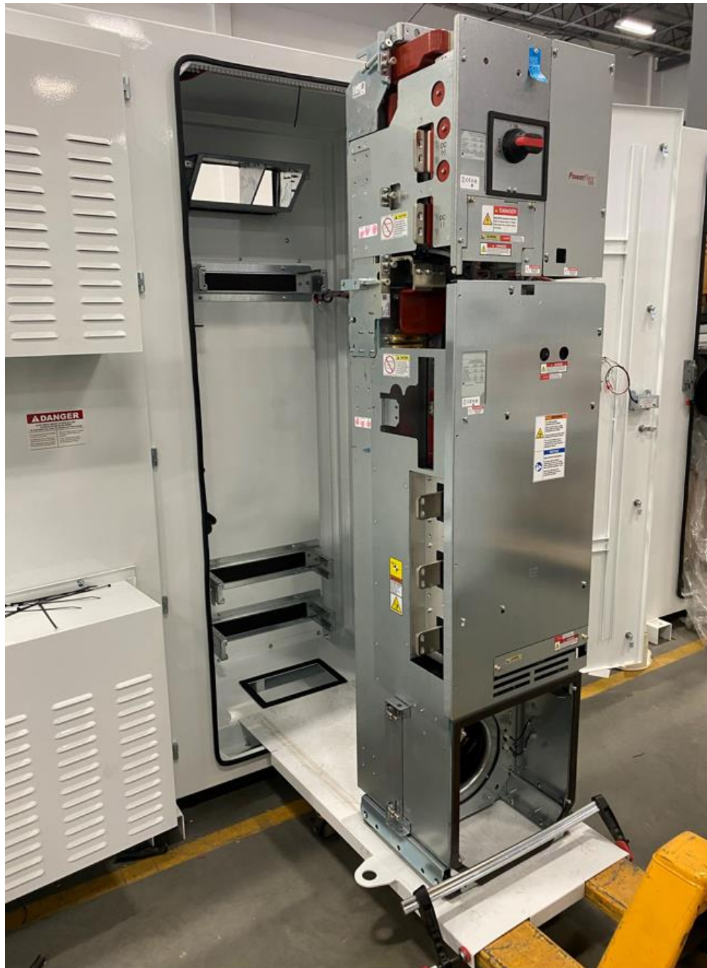
Figure 4-10: Module Placed on the Roll Out Cart
